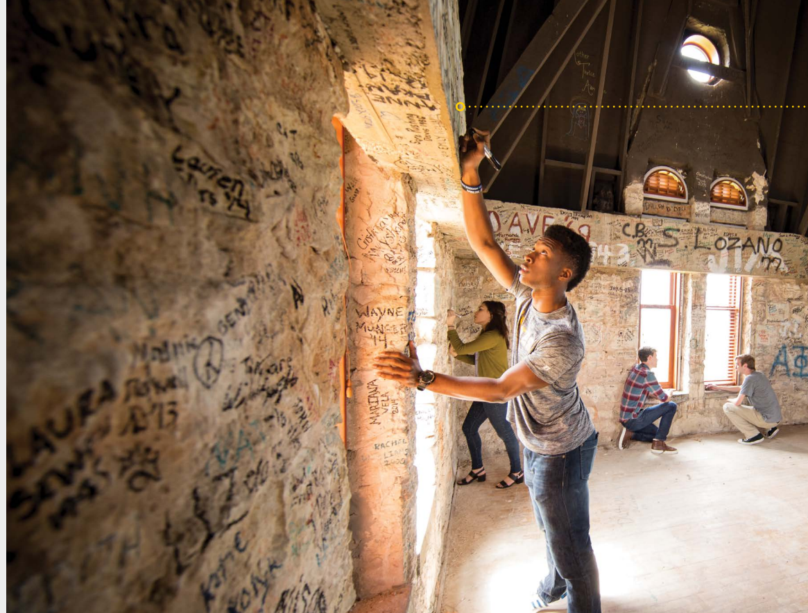
FOR MORE THAN A CENTURY, GRADUATING SENIORS HAVE ASCENDED THE HIDDEN STAIRCASE WITHIN THE CULLEN TOWER TO SIGN THEIR NAMES ALONG ITS WALLS.
